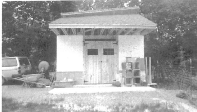
Image 1. Structure is built on a cement pad and has a stucco and stone finish
