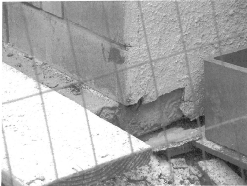
Image 5. Structure is built on concrete slab and not moveable
