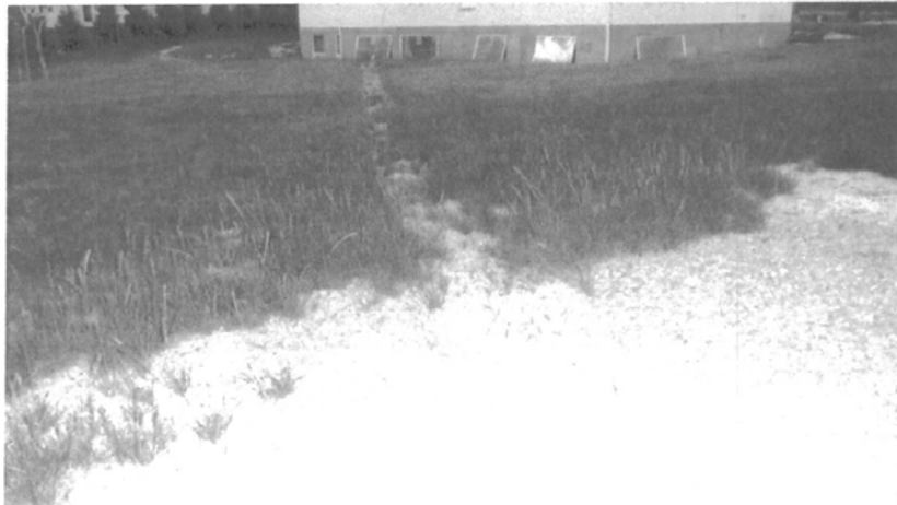
Image 7. Trench from house to accessory structure for power
